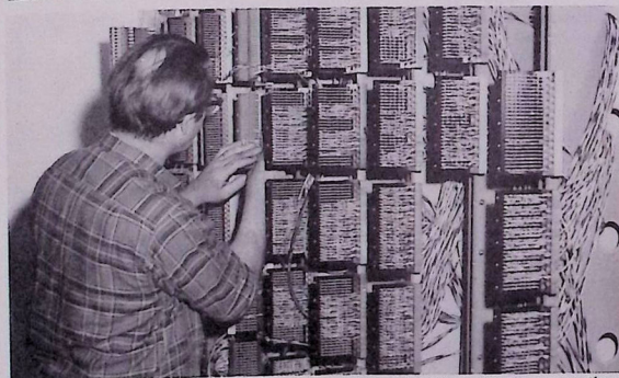
Mr. Keith Forsyth of Sask. Tel Moose Jaw, checking circuit connections for the new automatic system.
