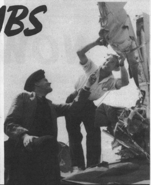
Aerial warfare roughed up this Mossie. Cpl Jerry Booton and FS R. C. Hector check woodwork damage.
