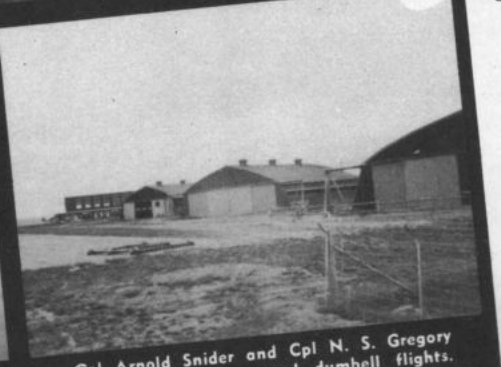
Saddle horses and stored equipment have replaced planes in old-style hangars.
