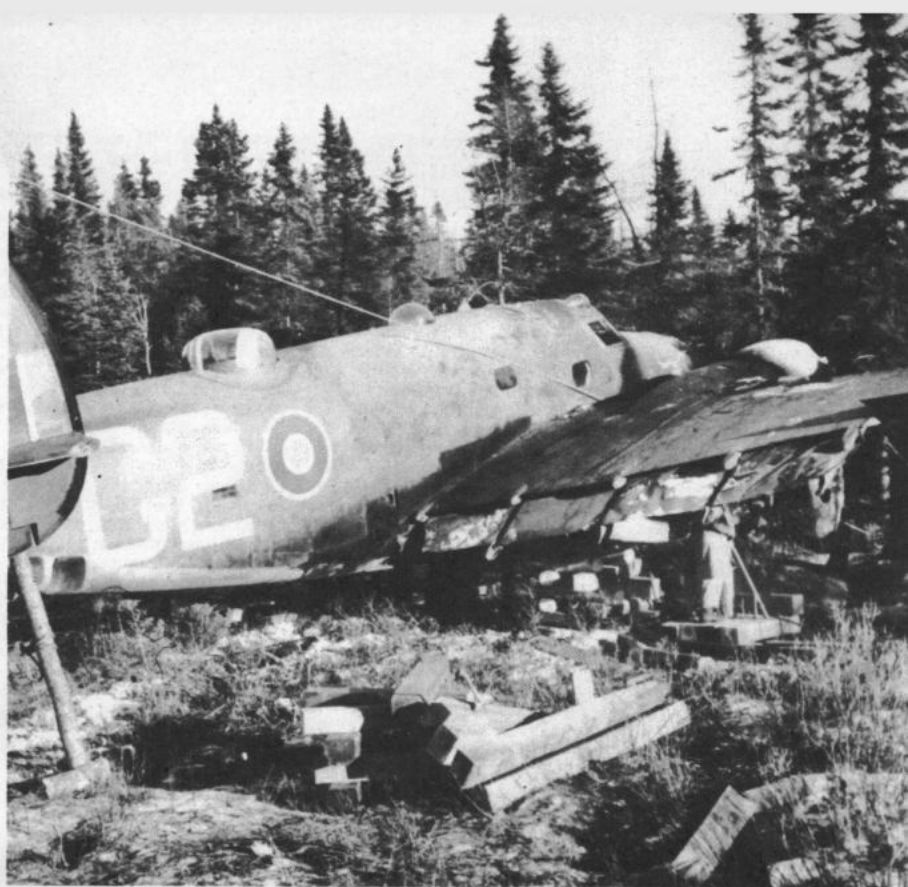
VENTURA SPLIT ITS NOSE IN PILE-UP BUT MECHS SOON HAD IT AIRWORTHY
