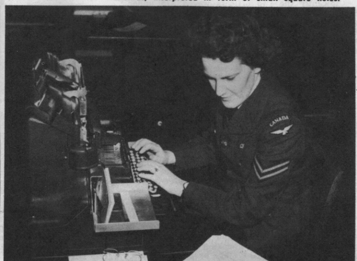
Cpl Eileen Moore, Saskatoon, runs complicated machine transferring info from "DRO's" to cards, interpreted in form of small square holes.
