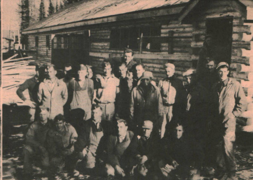
No. 4 CMU works and buildings section needed accommodation at Watson Lake in a hurry so these RCAF crewmen whipped this building into shape.
