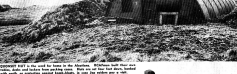
QUONSET HUT is the word for home in the Aleutians. SCAFOS built their own tables, desks and lockers from packing cases. Heat on hot feet down, hunked with earth, as protection against bomb-blasts, in case Jap cadets pay a visit.
