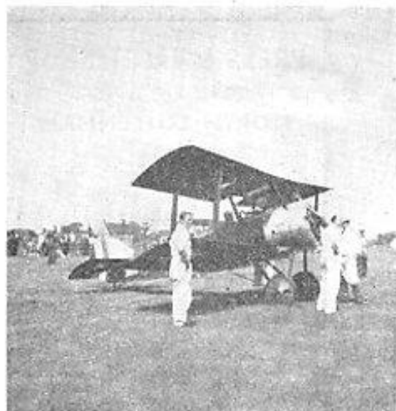
LEFT —Sopwith Pup (80 h.p. Le Rhone) single-seat scout biplane of 1915; used extensively by R.F.C. and R.N.A.S. Carried machine-gun firing ahead through airscrew disc. Span: 38 ft. 9 ins. Unable to compare performance with Luffenham's Sabres as data unavailable.
