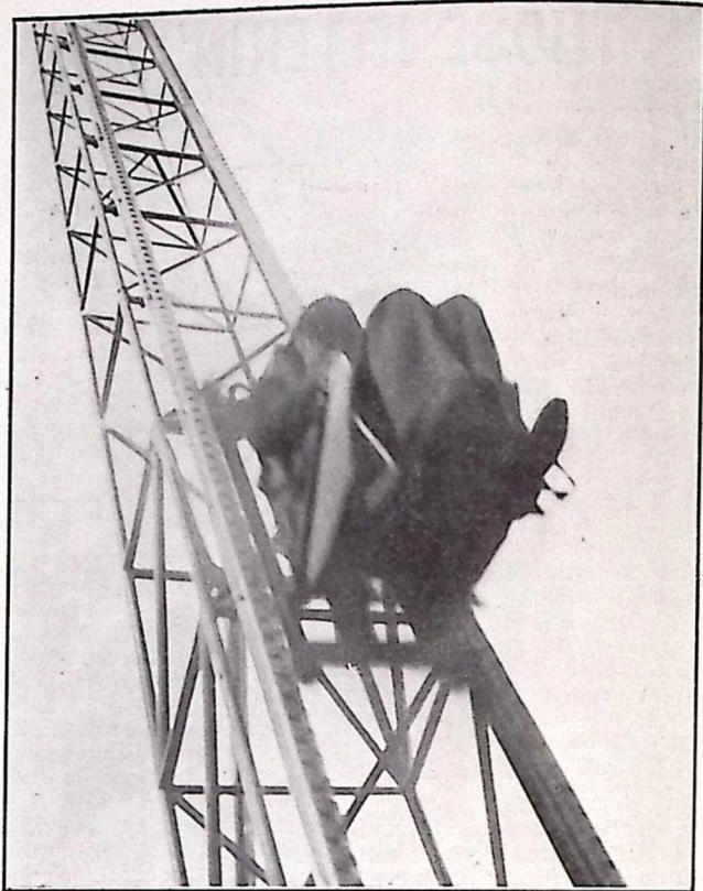
A few weeks ago a rather queer looking contraption arrived at RCAF Station, North Luffenham, something vaguely resembling a firemen's ladder. It was an ejection seat, complete with live cartridges, mounted on a 50 ft. rail, which in turn is mounted on a trailer truck. A large number of No. 1 (F) Wing personnel were checked out. It is the quickest checkout known. You climb aboard untrained, pull a curtain over your face and are sitting 35 to 40 feet up the rail, fully trained. Seen in the above photo is C/C E. B. Hale halfway through his training.
