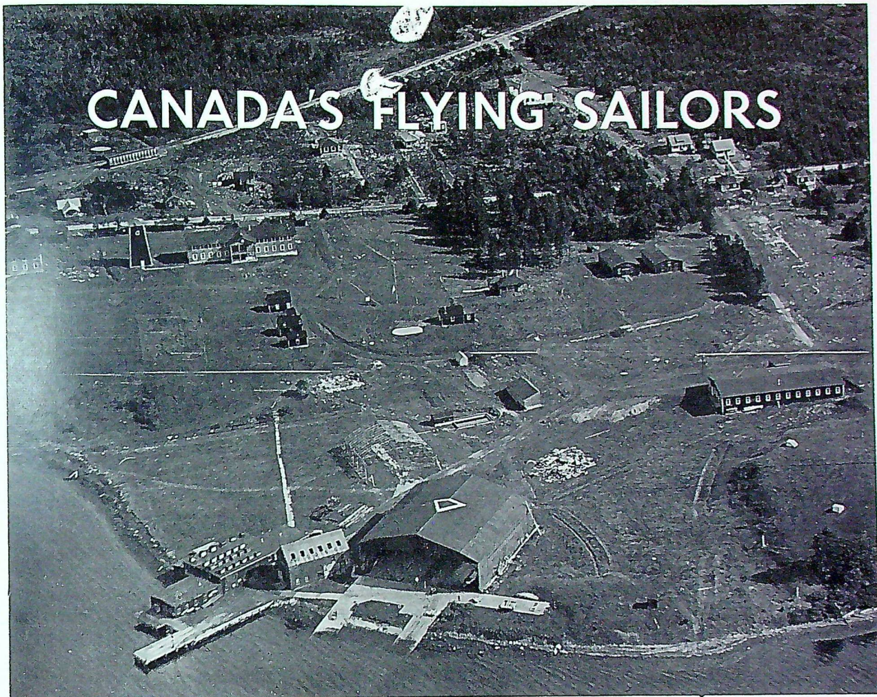
Dartmouth Air Station, 1920.
