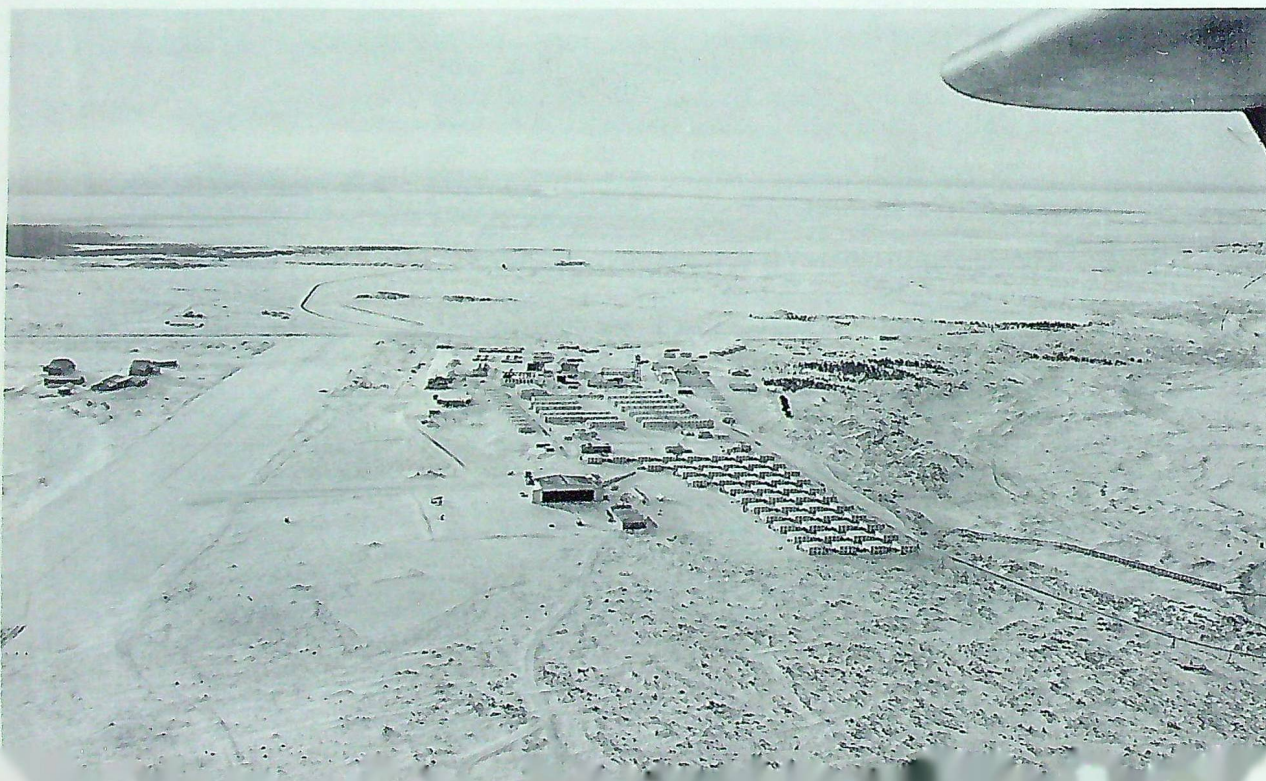
RCAF turned over Churchill aerodrome control and other facilities (such as hangar in centre foreground) to DOT this spring.
