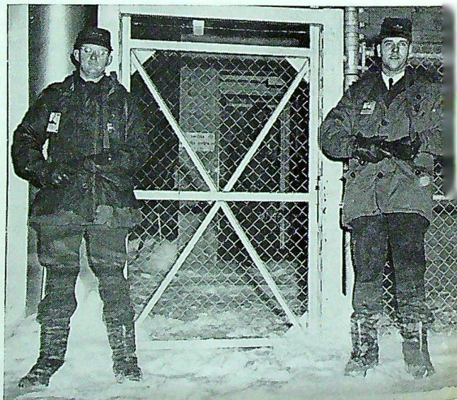
RCAF security guards, carbines at-the-ready, guard the Bomarc storage facilities at North Bay, Ontario.
