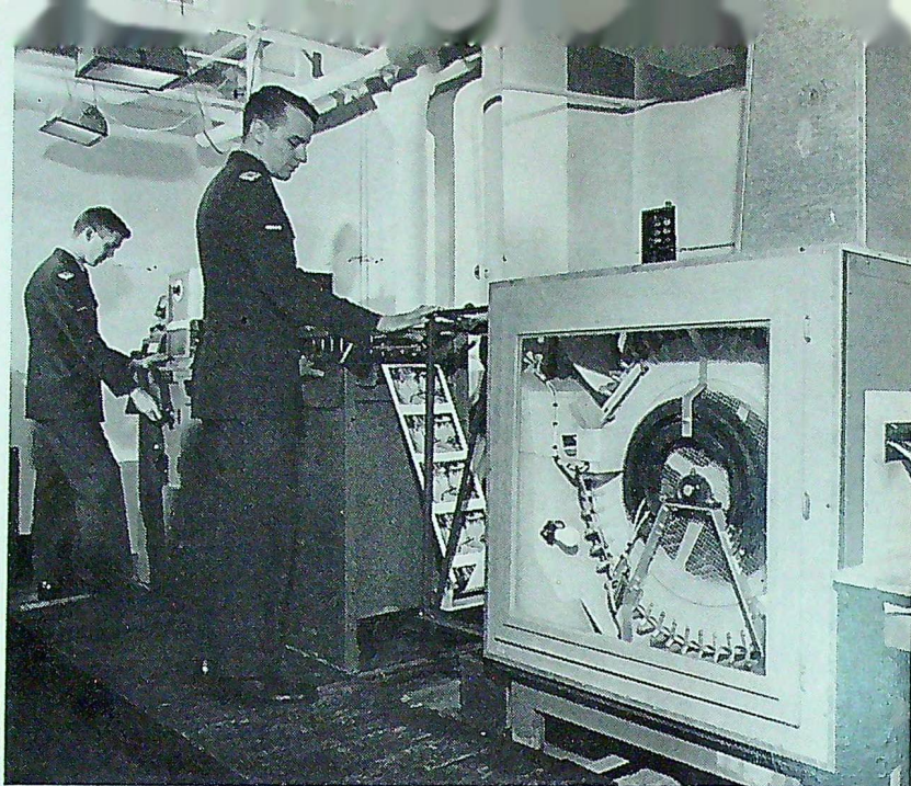
Volume printing, developing, washing and drying from a single negative onto 1000-ft. strips of sensitized paper are accomplished uniformly by this multi-printer.
