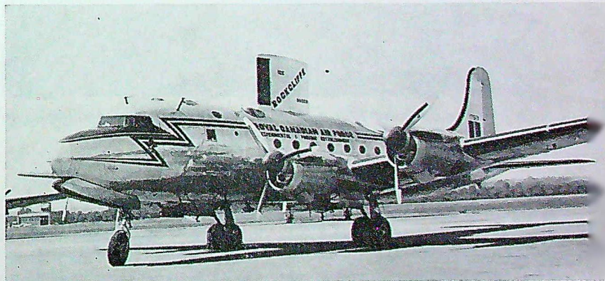
"Rockcliffe Ice Wagon", a modified North Star used by CEPE to study ice accretion in the early 50s.
