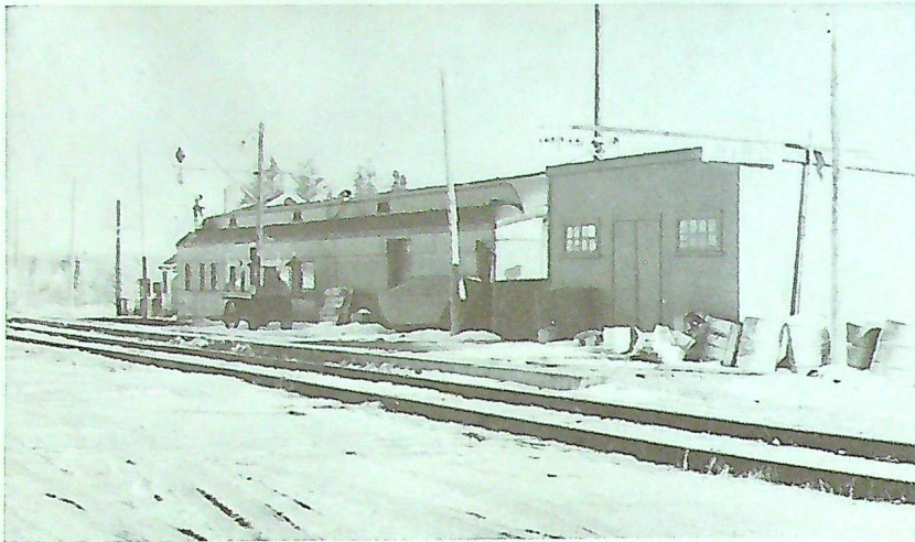
Improvised railway station between The Pas and Churchill.
