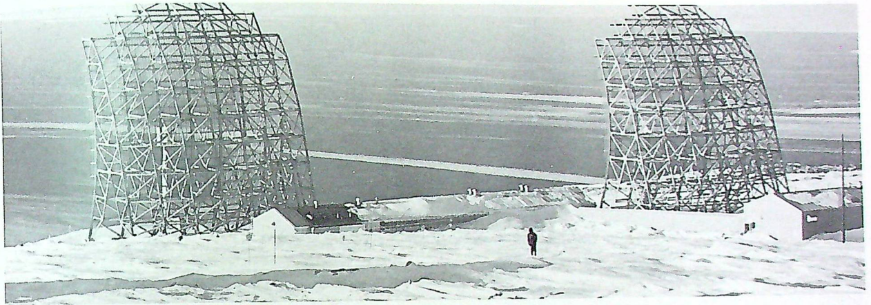
Rearward communications antennae at Cape Dyer in Canadian Arctic
