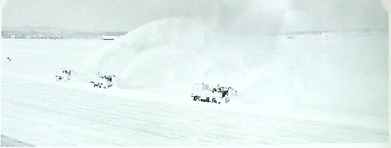
Year-round aerodrome maintenance necessitates modern snow-removal equipment
