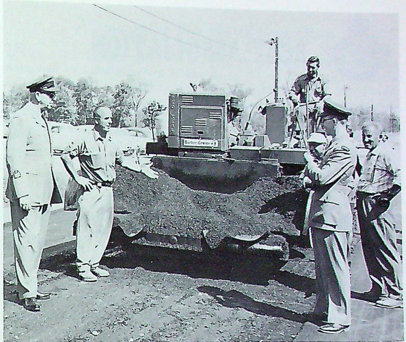
WO Fleming here gives assistance in inspection of work on a road contract to F/O C. T. Harnden who is responsible for co-ordinating the supervision of contracts.
