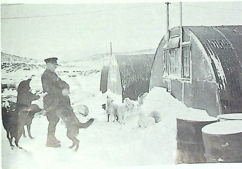
At No. 30 R.D., Cape Bauld, Nfld.
