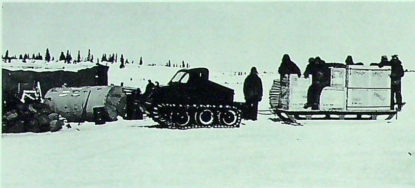
Bombardier tractors hauled equipment from lakehead landing sites to construction points.
