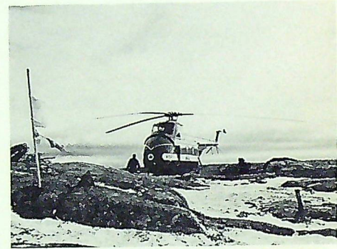
An R.C.A.F. helicopter being unloaded on a rocky hill-top where one of the Mid-Canada Line's detection-stations will stand. (Photograph by Cpl. Darrel Eagles, A.T.C.H.Q.)
