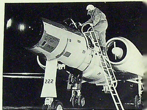
When towing targets for practice firing, this CF-100 is rendered clearly visible by its coat of fluorescent red paint.
