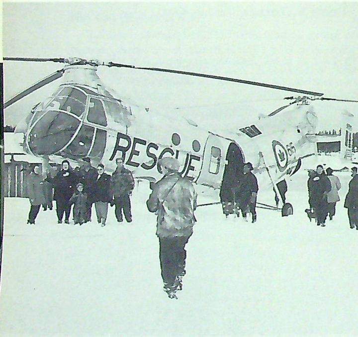
Landing at Lake Manuan dam site.
