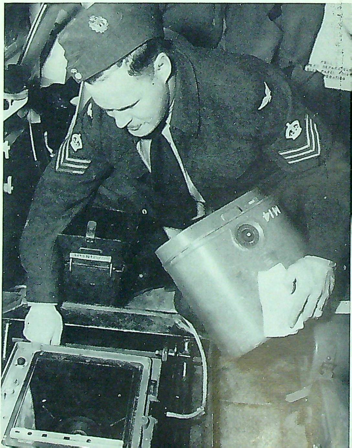
Flt. Sgt. W. G. Brannon checks the survey camera between lines.
