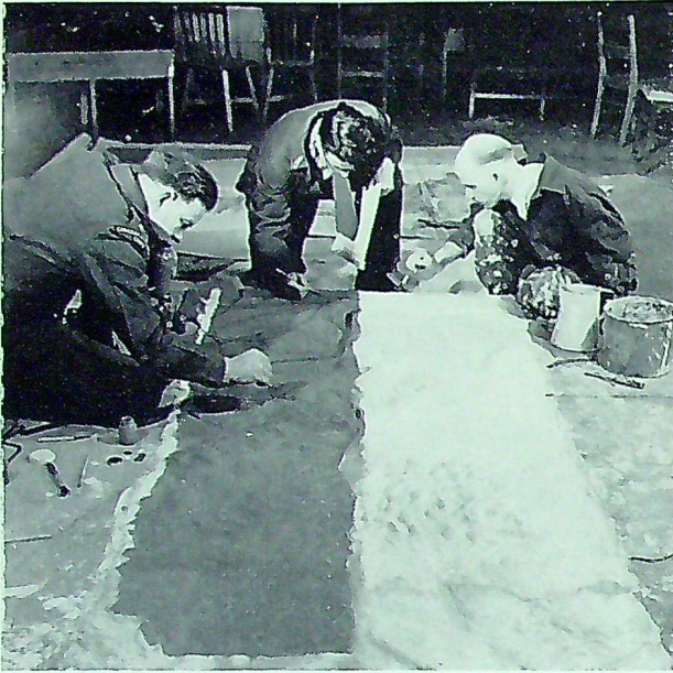
Shading and plastering.
