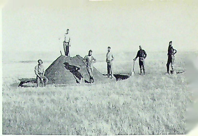
Royal Engineers building boundary mound.
