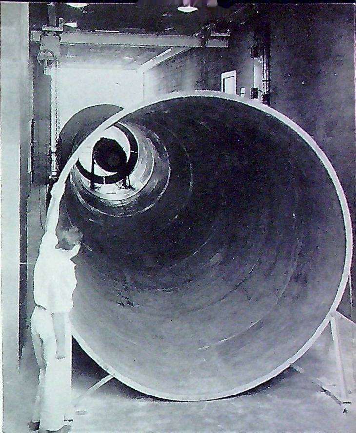
Exit end of ejector tunnel
