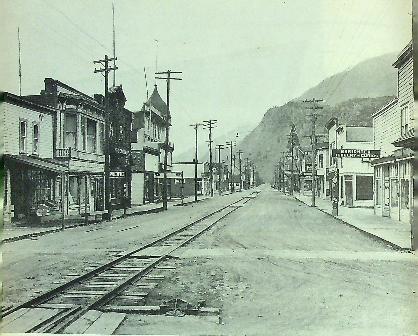
Main Street, Skagway. W.P. & Y.R. tracks in centre
