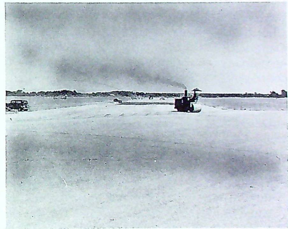
The runways at Pendleton nearing completion.
