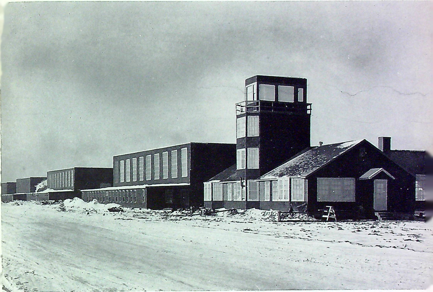
The Control Tower at No. 8 S.F.T.S. Moncton, N.B.
