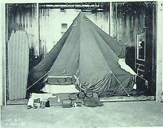
Camping in Cold Chamber to test personnel equipment
