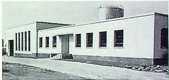
Low Temperature Laboratory Building
