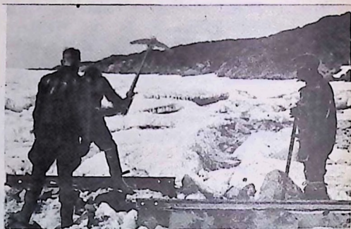
Laying track at foot of slipway: Nottingham Is.
