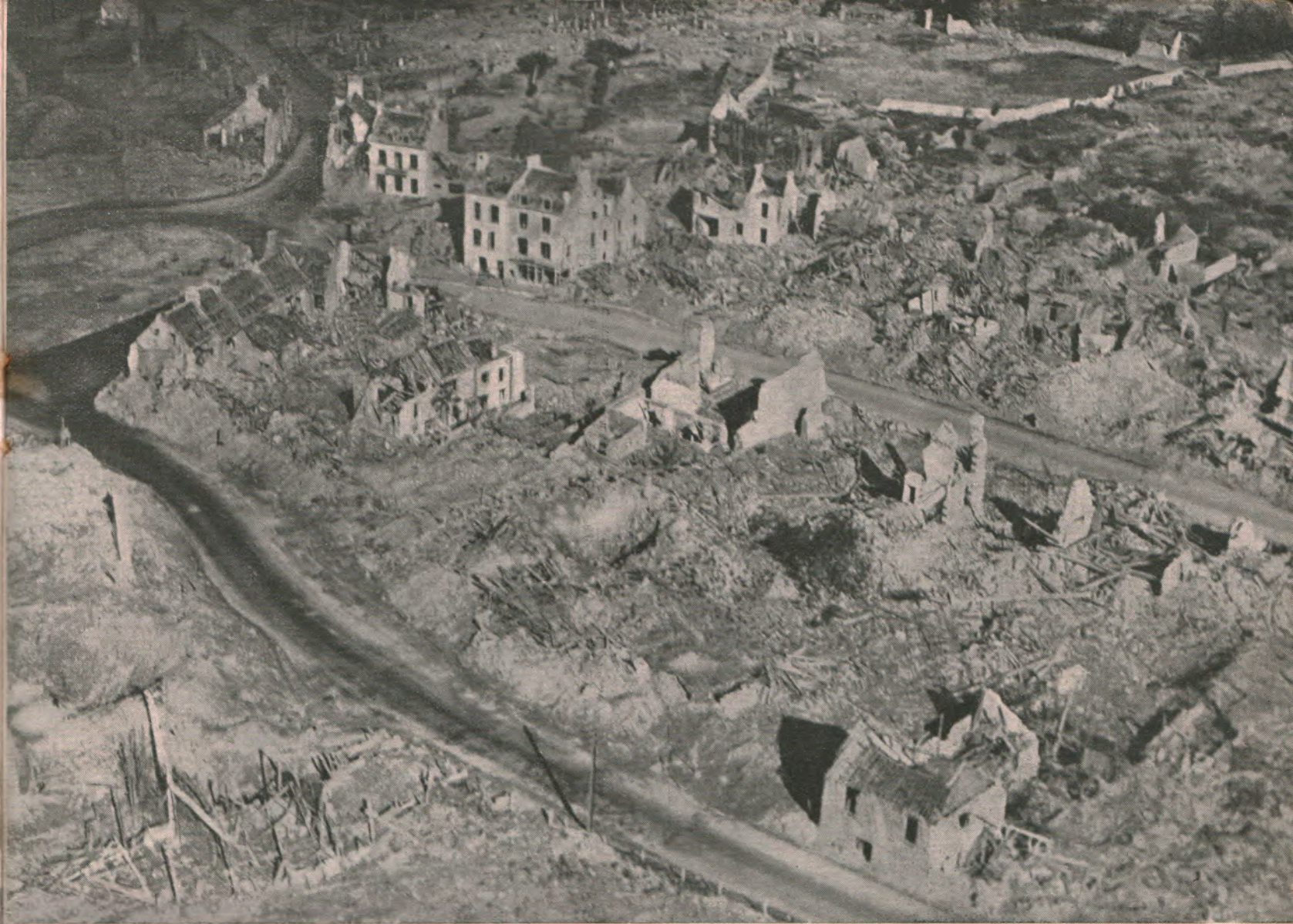
". . . . The desolation of Villers Bocage".
