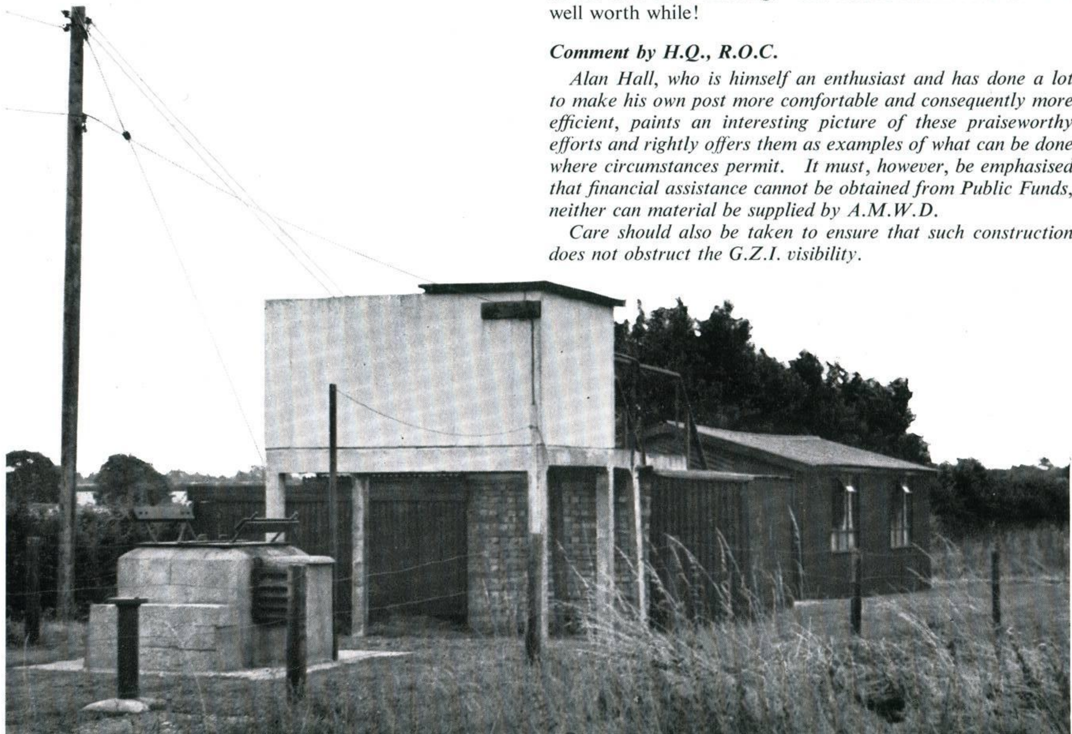
A general view of the 4/L2 Little Waltham post site.
