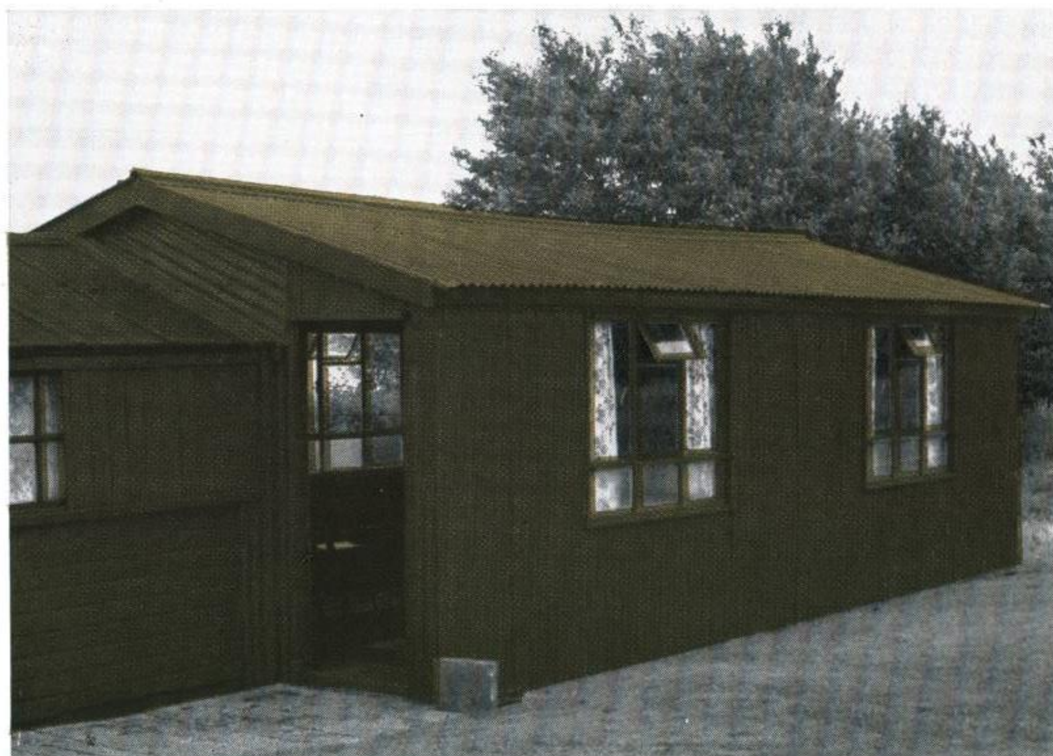
"Dane's Hall," 35 feet long, built from wooden framing and clad in corrugated iron.
