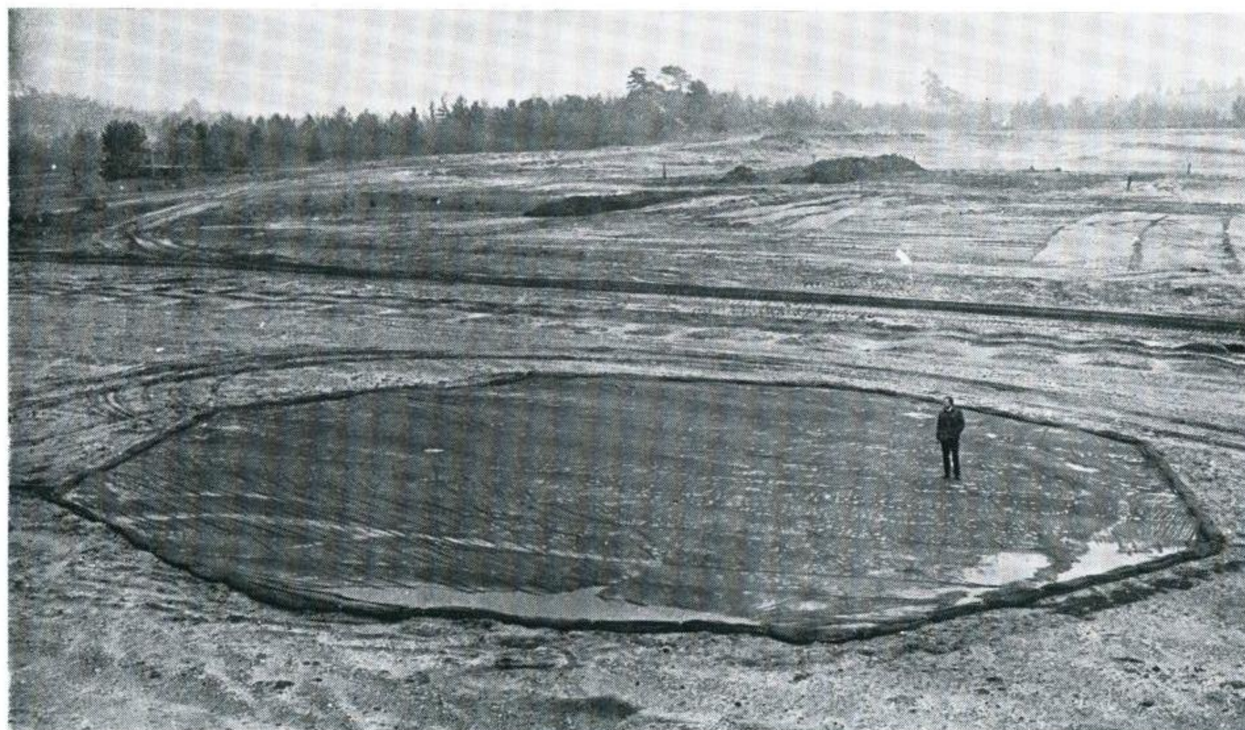
One of the two prototype ultra-light helicopter membranes which has successfully undergone trials at the Joint Helicopter Development Unit, and is being tested in NW Europe.
