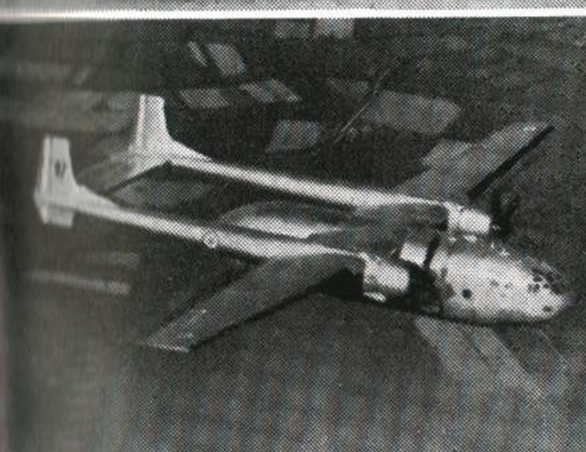
NORATLAS (FRANCE) Military Transport Wing-tip heater fairings not always fitted. Span: 107 ft.
