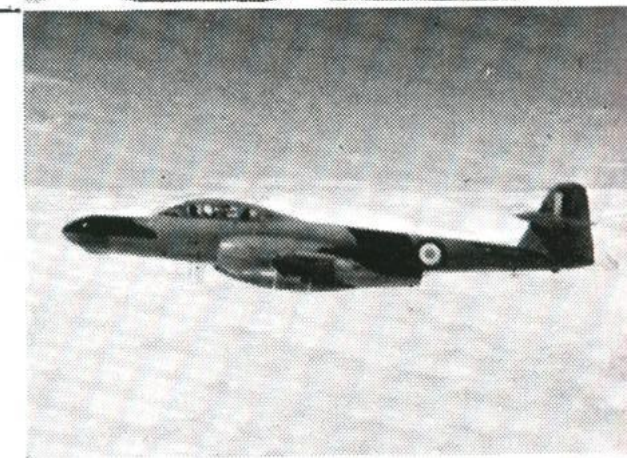
METEOR NF Mk. 11 (G.B.) Night Fighter Ventral fuselage and/or under-wing tanks may be carried. Span: 43 ft.
