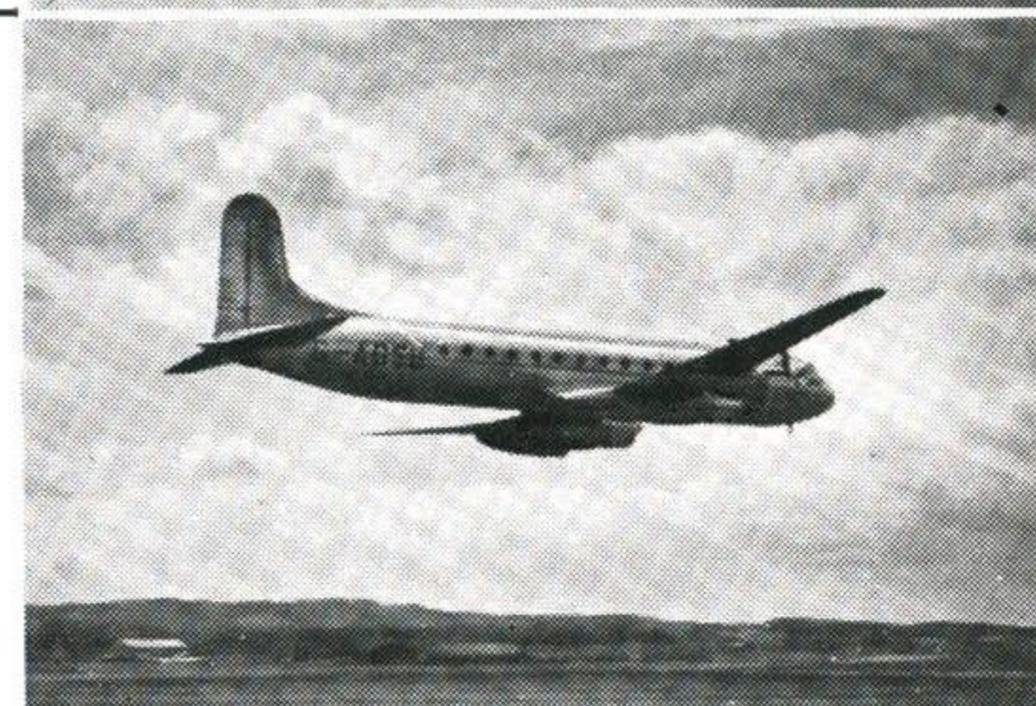
Avro TUDOR 2 (Four Merlin 621 engines) Span 120' 0" Length 106' 7" (Tudor 5 is the same except for circular windows)
