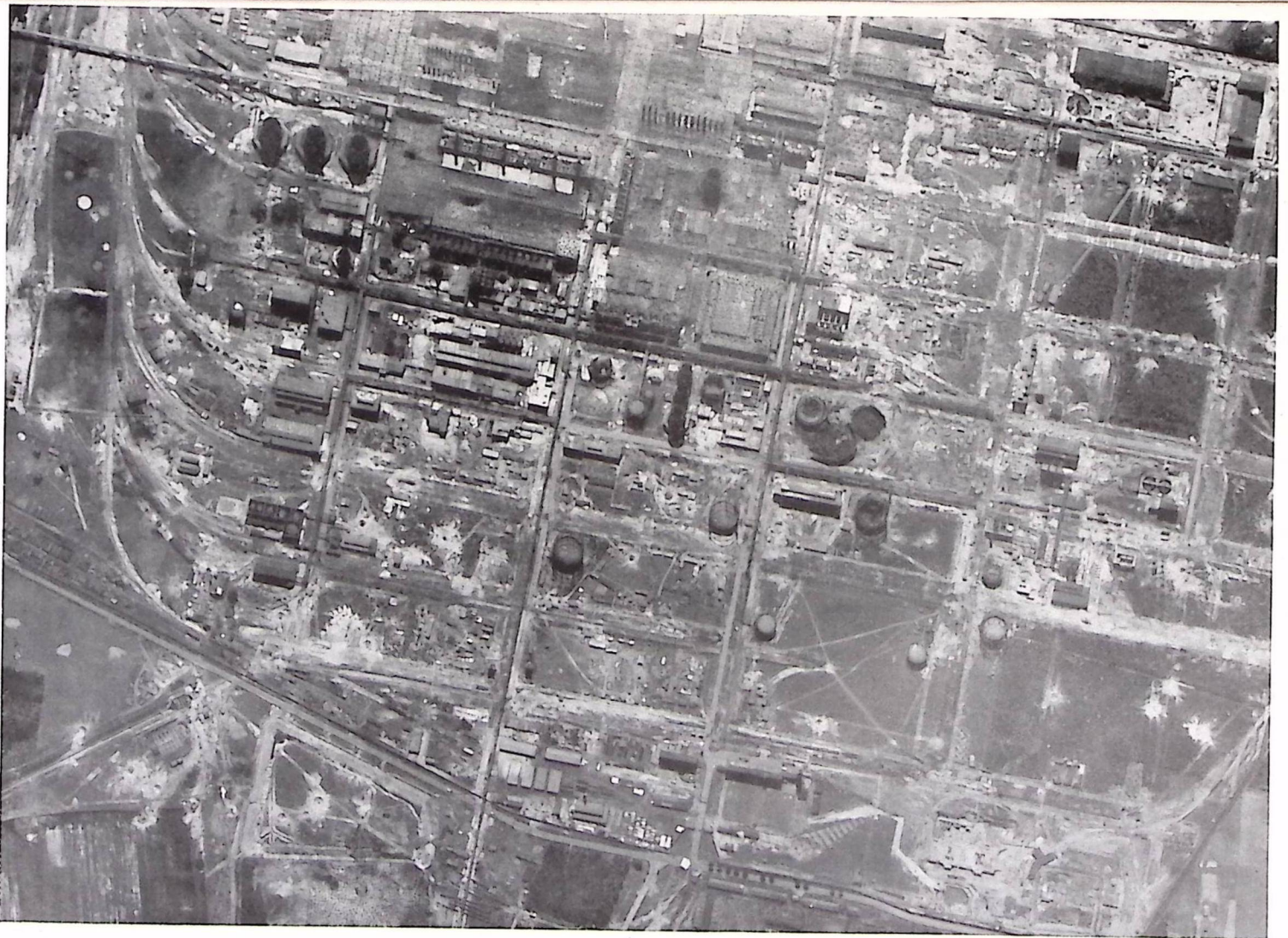
Extensive damage was caused in the U.S.B.C. daylight attack (22.6.43) on the important Synthetic Rubber Works at HULS, N.W. of Krefeld. This plant, the second of its kind in Germany, was built in 1940 as an addition to the existing plant which was producing ethylene glycol. Many of the most important plants and buildings were damaged in the attack and it is considered that the plant will be out of production for at least four to five months. Six gas holders were destroyed.
