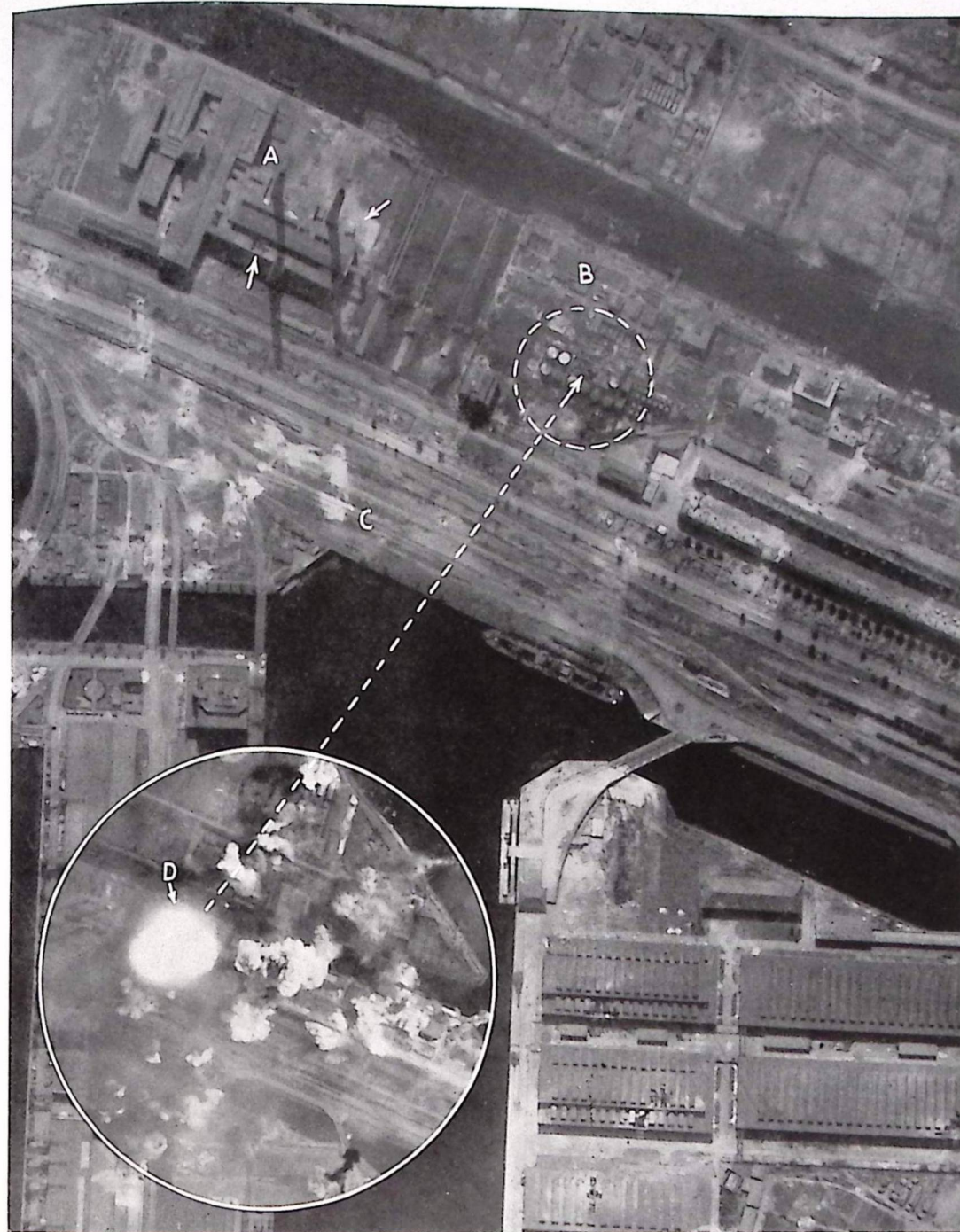
The Neuhoef Thermal Electric Power Station (A), one of the largest and most important in HAMBURG, was damaged during the attacks. The Hansa Mühle Seed Crushing Plant (B) has been considerably damaged, storage tanks being demolished. There are a number of craters on the railway sidings (C). INSET: An explosion (D) indicating that the oil storage tanks were hit during the U.S.B.C. attack on 25.7.43.
