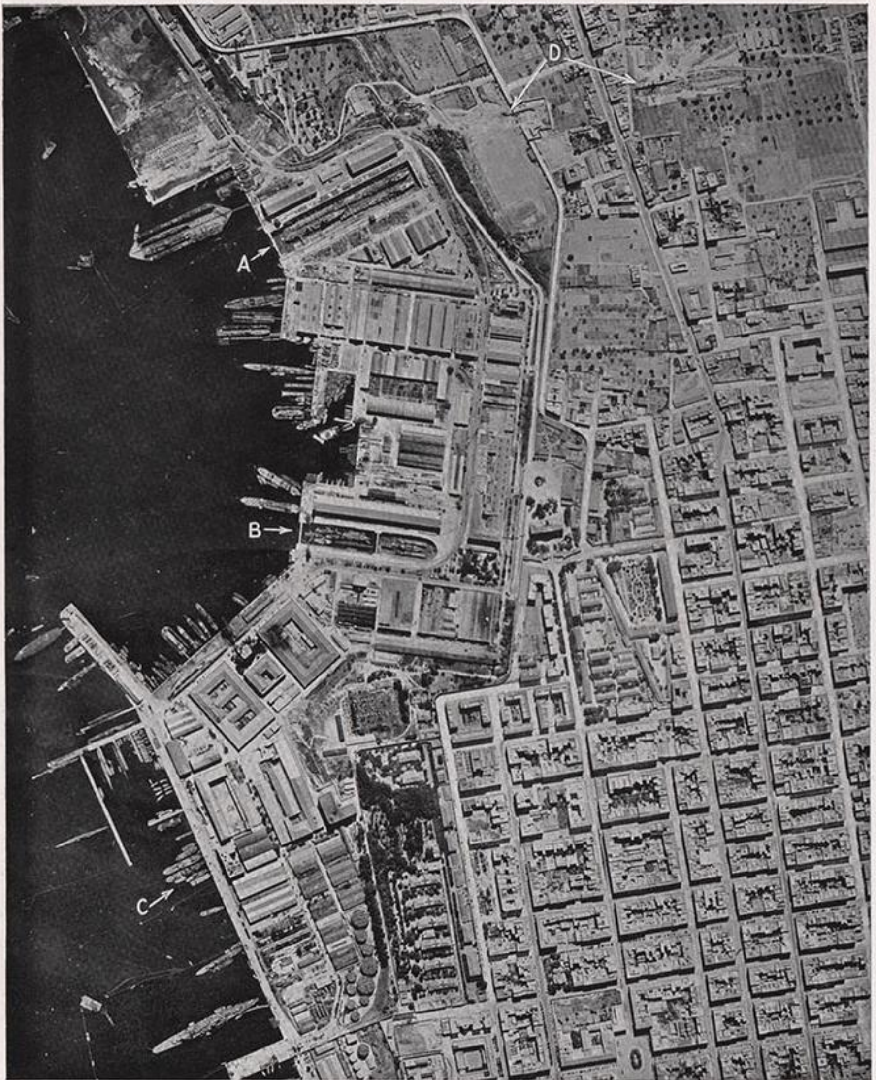
Minor repairs to naval units are carried out at the Naval Dockyard on the south shore of Mar Piccolo (West), TARANTO. The new Dry Dock (A) and Principe di Napoli Dry Dock (B) are used to accommodate all types of naval ships and large merchant vessels. The Submarine Base (C) is also used by major naval vessels. A tunnel is being cut from the Dockyard towards a large dry dock under construction in the Mar Grande (see next page). Excavations are seen in progress at two points (D).
