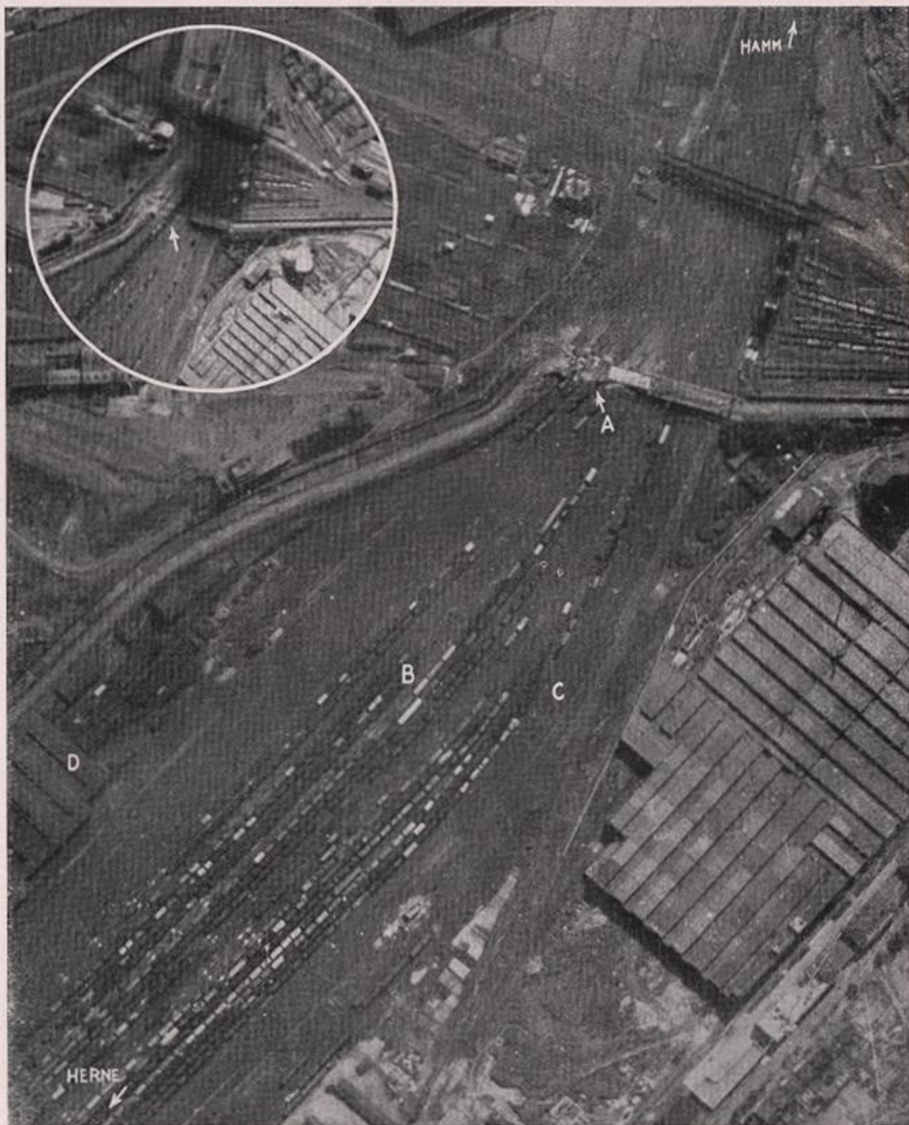
Five days after the attack on DORTMUND on 23/24.5.43 the eastern span (A) of the bridge carrying the Westfalla Strasse over the entrance to the main marshalling yard is seen collapsed as a result of a hit. It is obstructing all but three of the roads from the south into the yard (B) and would stop the working of traffic through the yard in a northerly direction. (C) Through lines. (D) Locomotive Depot. Inset: Damaged bridge being cleared away.
