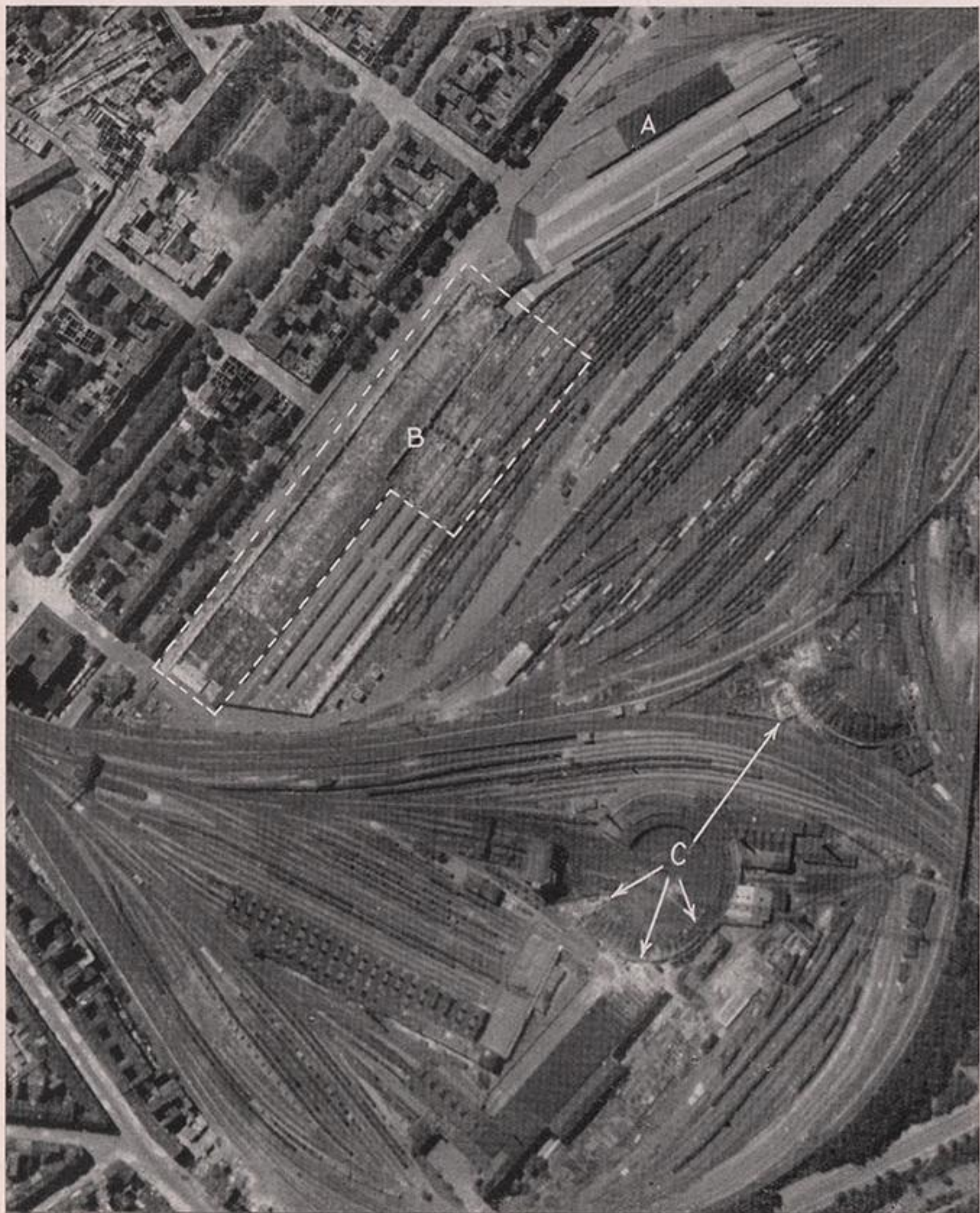
In early 1942 sheds which occupied the site (A) at the Gereon Goods Depot, COLOGNE, were severely damaged and the sheds were rebuilt to a simpler plan. (See page 19, Vol. 3, No. 1.) In the recent attacks 75 per cent. of the adjoining buildings (B) were destroyed. Considerable damage was also caused to the Engine Sheds and other buildings (C) attached to the railway sidings.
