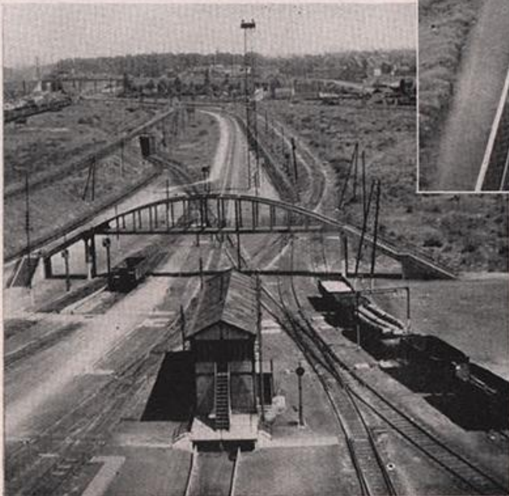
The northern end of LILLE/LA DELIVERANCE Marshalling Yard with mixed goods stock in the forwarding sidings (foreground). The reception sidings and locomotive engine sheds are to the left middle distance.
