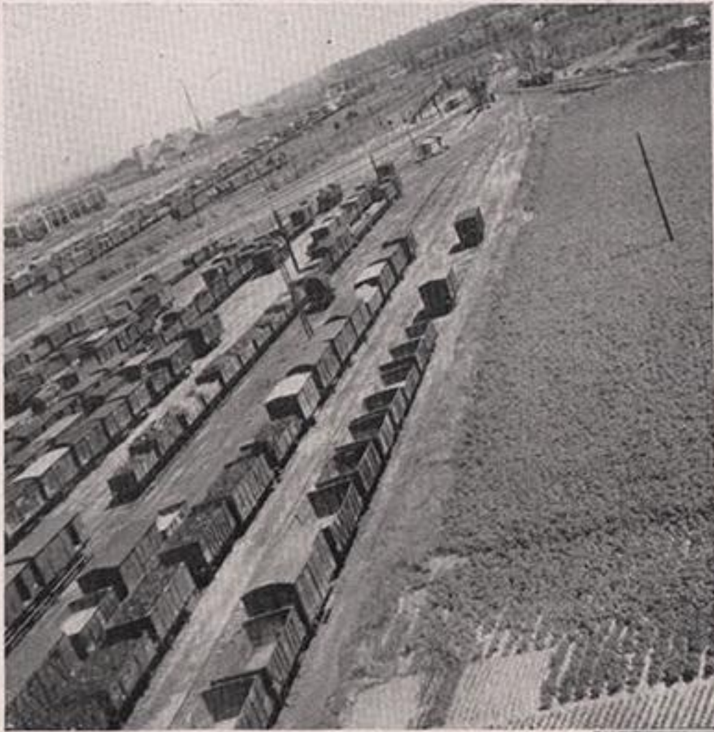
The northern end of LILLE/LA DELIVERANCE Marshalling Yard with mixed goods stock in the forwarding sidings (foreground). The reception sidings and locomotive engine sheds are to the left middle distance.
