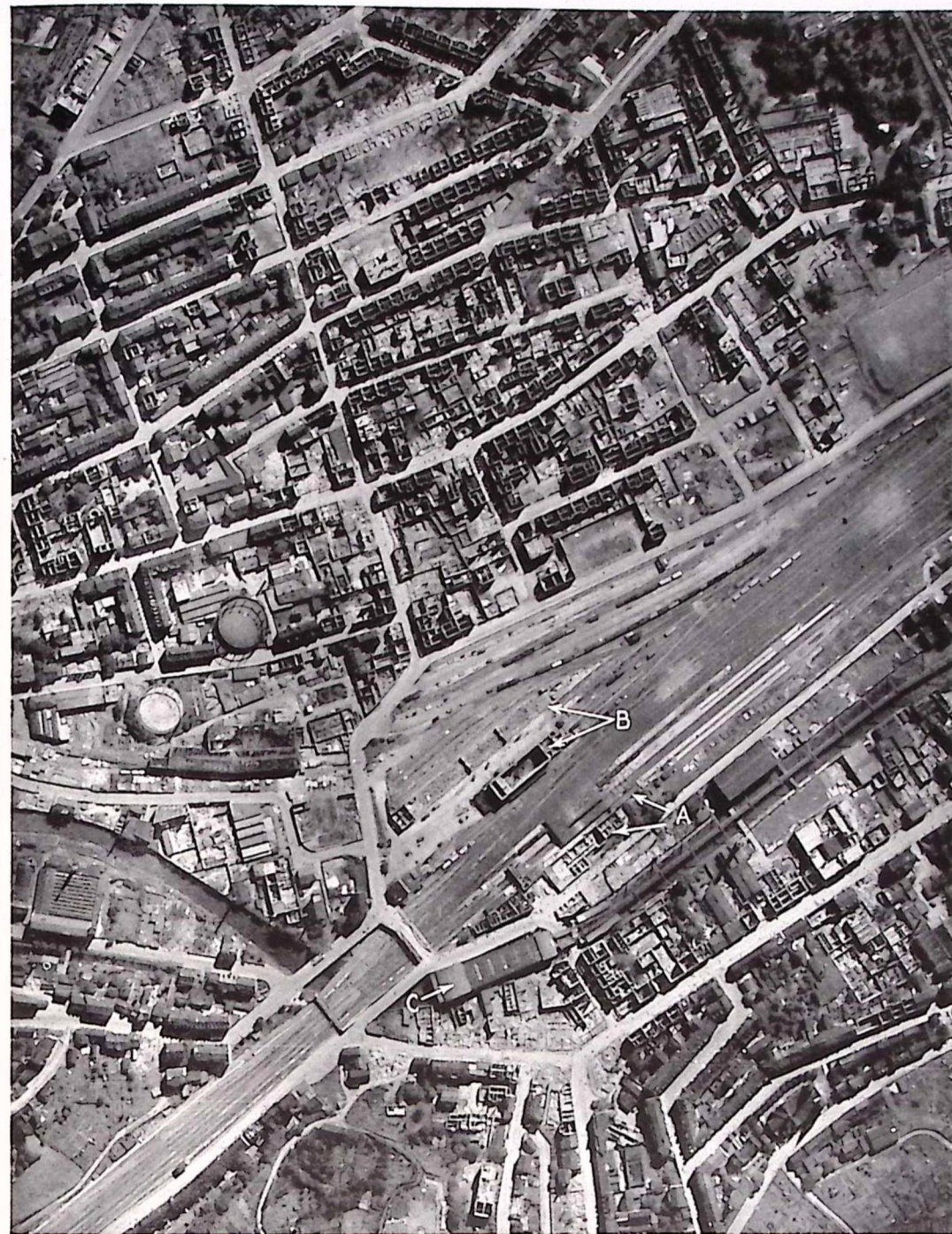
BARMEN-RITTERSHAUSEN Railway Station was devastated. The Passenger Station (A) and Goods Station (B) have been wrecked and numerous small factories are included in this large area of destruction. The terminus of the Overhead Railway (C) is surrounded by the shells of buildings.
