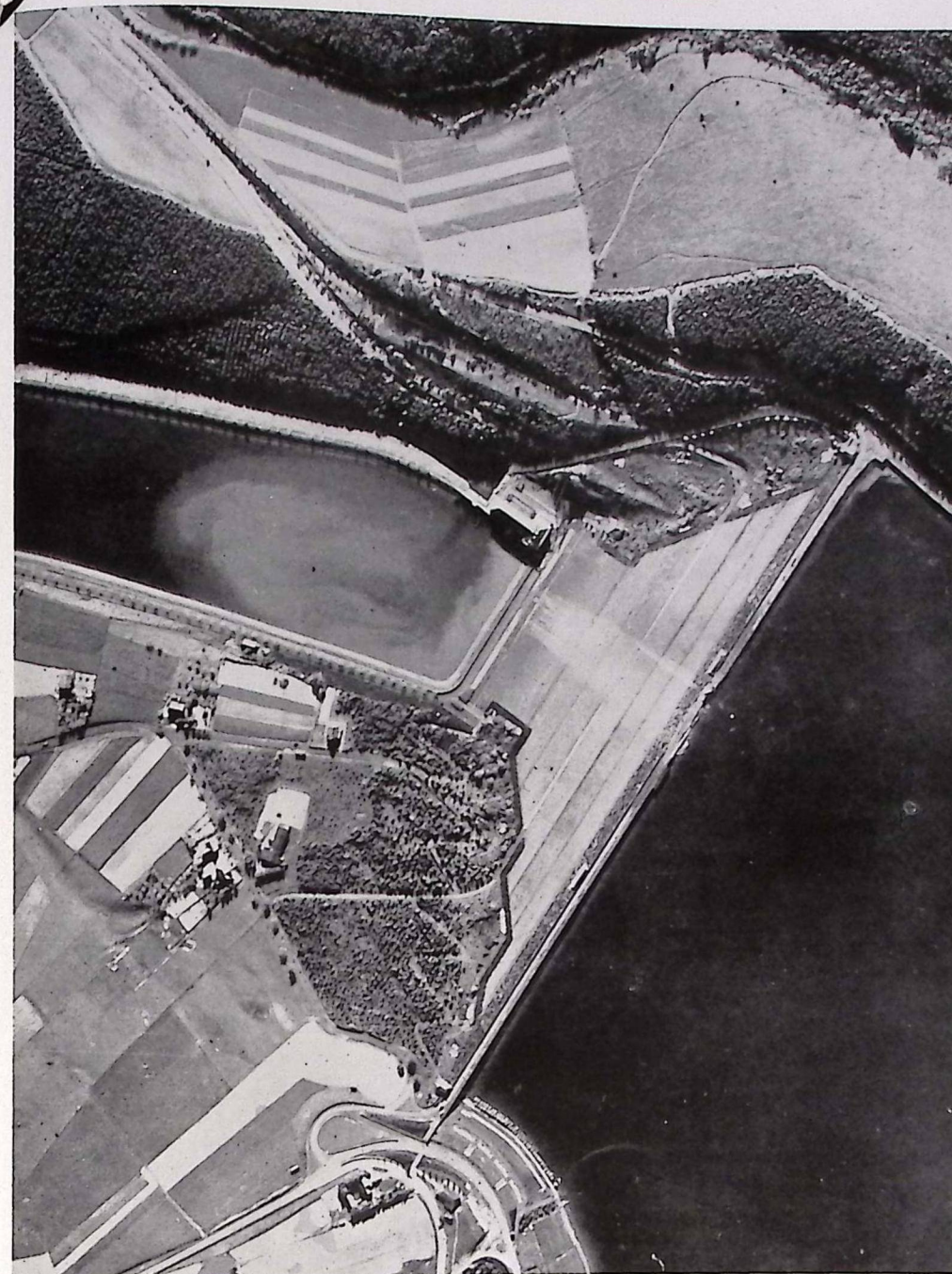
A stretch of about 200 ft. on the crown of the SORPE DAM was damaged during the night's attack (16/17.5.43). Water appears to have run down the face of the dam and has carried earth from the dam into the Compensating Basin.
