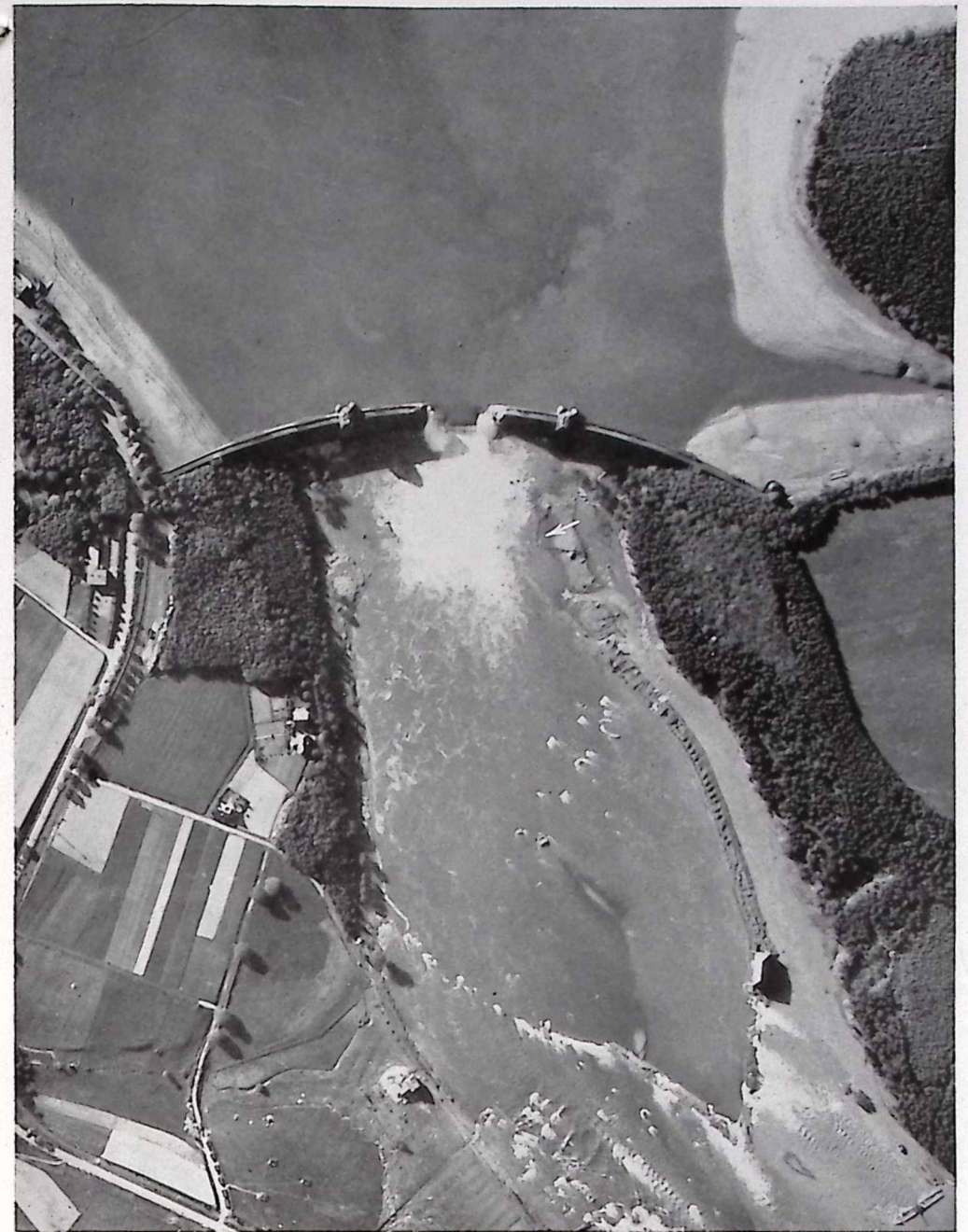
The bombers made a breach of about 240 ft. width in the Moehne Dam. When this photograph was taken several hours after the attack water was still flowing through solid. Turbulent water and foam cover the site of the Power Station destroyed in the flood. The dam surrounding the Compensating Basin has been destroyed and houses and farms washed away in the flood of water. Note the remains of the torpedo boom (arrow).
