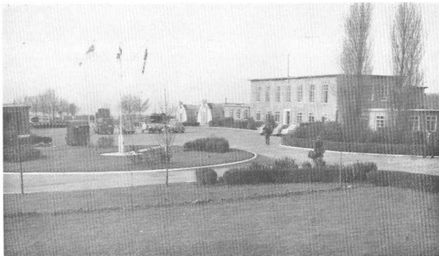
Administration Building and Main Gate
