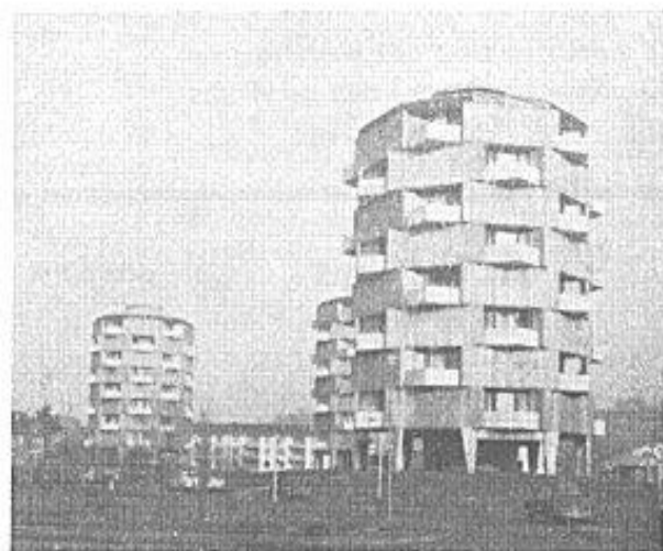
PMQ — «TOWER APTS» — 8 stories (with elevator) 8/1 bedroom and 16/2 bedroom Apts in each building.
