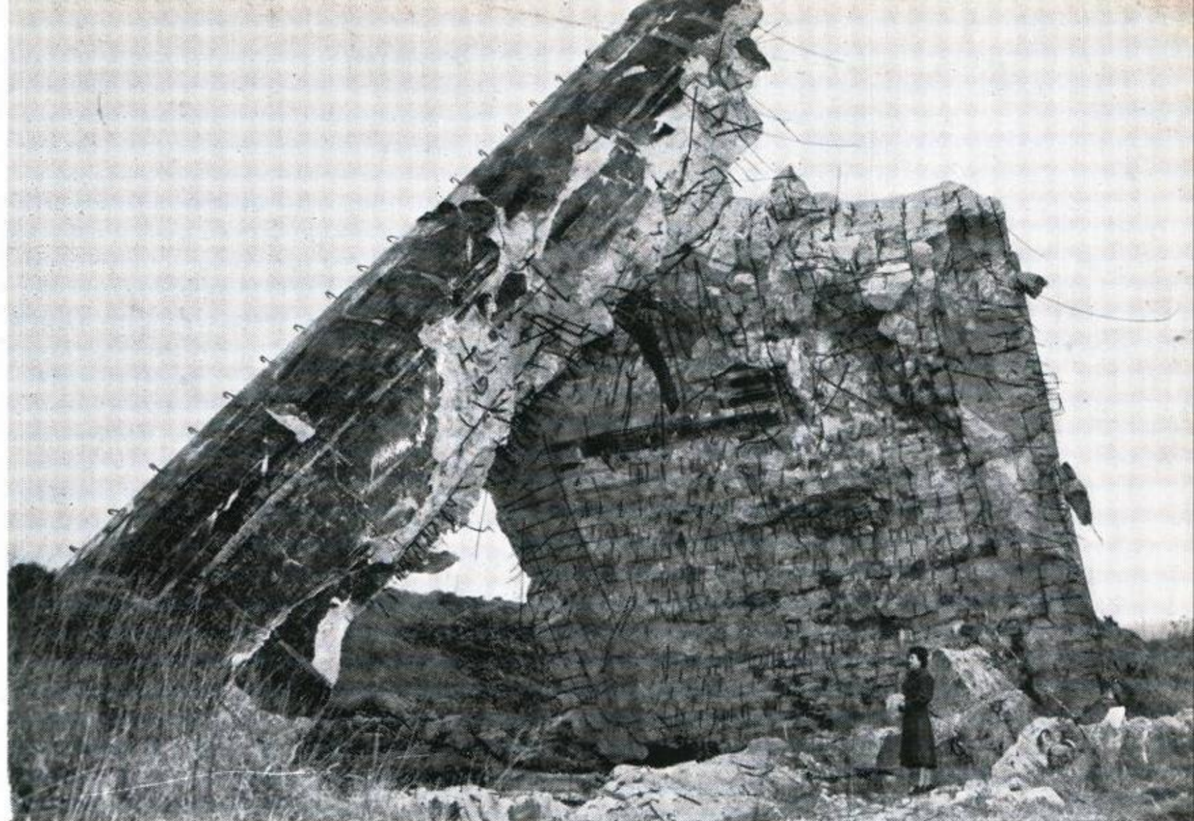
Some idea of the size of this demolished bunker can be gauged from the airwoman standing in the bottom right hand corner of the photograph. It stands in the middle of a farmer's field, a few hundred yards from the airfield boundary fence.
