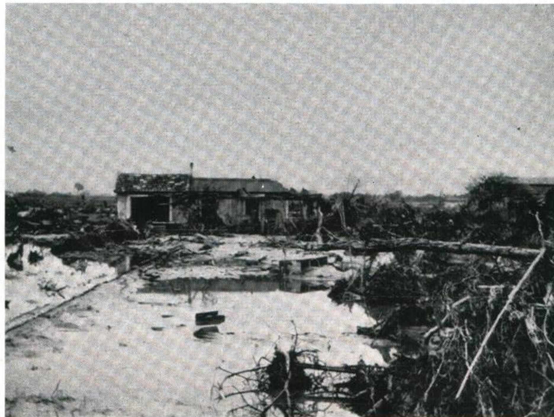
Frejus after the dam break.
