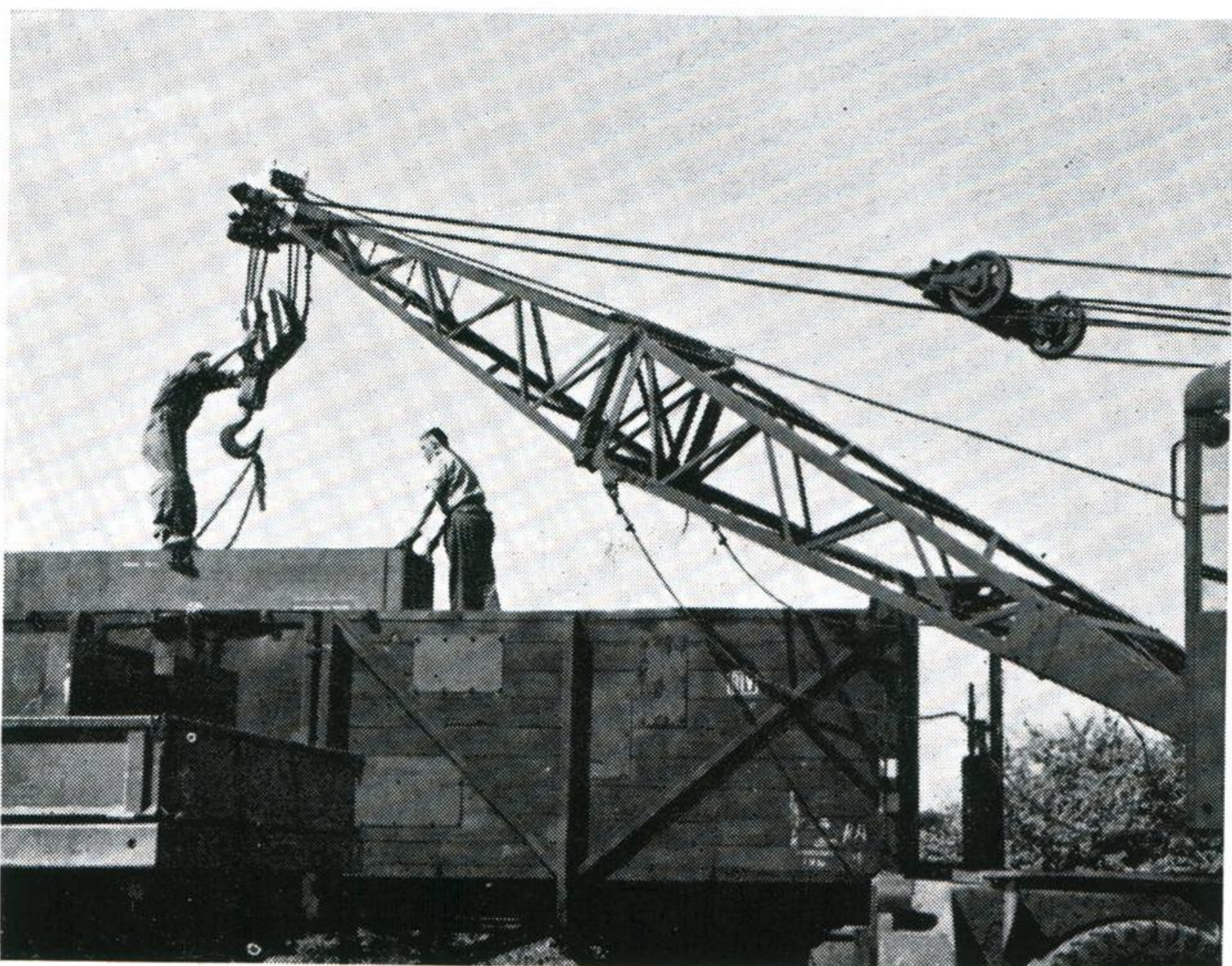
R & I personnel unloading material at Wintersdorf rail siding
