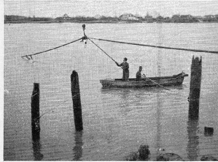
Aquatic linesmen — one bends on the oars as his pal "chisels" away at the snatch block. They both scam as the cable falls into the water.
