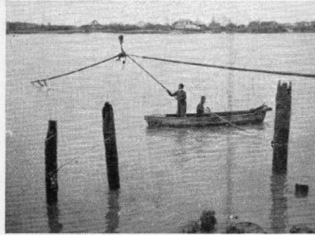
Aquatic linesmen — one bends on the oars as his pal "chisels" away at the snatch block. They both scam as the cable falls into the water.
