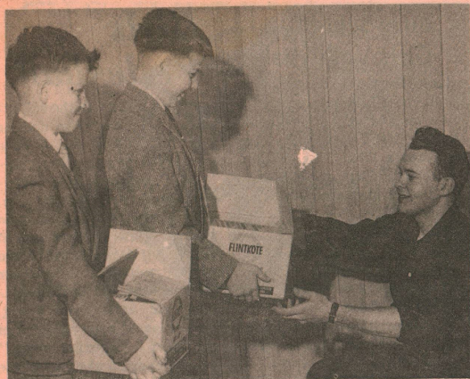
Brian Hodgins, (left), 12, and Bengt Forster, (center), also 12, lend a helping hand as Leading Aircraftman John Leduc, son of Mr. and Mrs. R. Leduc, 567 Mutual Street, Ottawa, begins laying a tile floor at the Brookdale Farm Children's Home, where the two boys are living. While the '33 children at the Wakefield, Que. home were attending an annual Christmas party sponsored by the Corporals' Club of RCAF Station Rockcliffe on Saturday, Dec. 17, LAC Leduc and thirteen other airmen put down a tile floor as a Christmas project. The money for the floor was collected from members of the Rockcliffe Airmen's Canteen.
