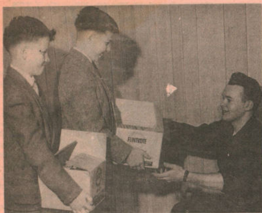
Brian Hodgins, (left), 12, and Bengt Forster, (center), also 12, lend a helping hand as Leading Aircraftman John Leduc, son of Mr. and Mrs. R. Leduc, 567 Mutual Street, Ottawa, begins laying a tile floor at the Brookdale-Farm Children's Home, where the two boys are living. While the 33 children at the Wakefield, Que. home were attending an annual Christmas party sponsored by the Corporals' Club of RCAF Station Rockcliffe on Saturday, Dec. 17, LAC Leduc and thirteen other airmen put down a tile floor as a Christmas project. The money for the floor was collected from members of the Rockcliffe Airmen's Canteen.
