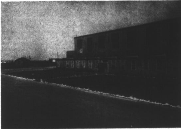
1st PRIZE—NO. 5 HANGAR
