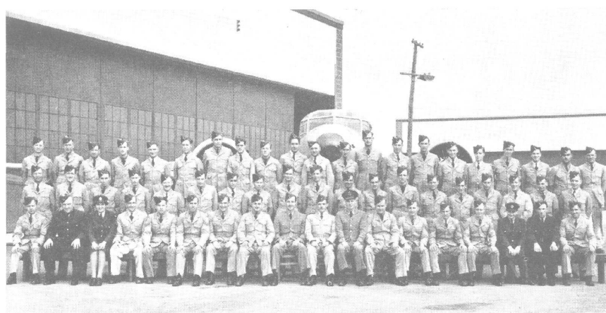
MINOR MAINTENANCE — R. C. A. F. STATION, MOUNTAIN VIEW
