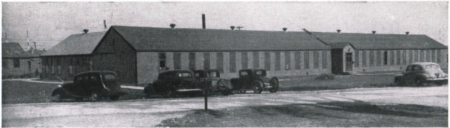
Main office building, where administration and pay offices are located.
